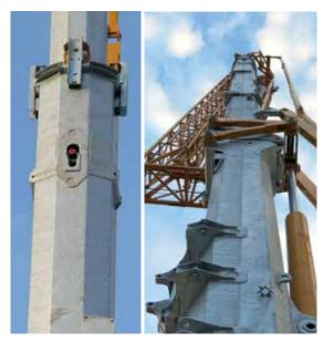
Automatic erection system requires no extra mast section to greatly reduce setup time
