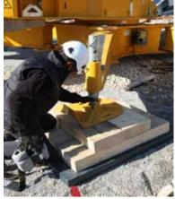
Quick and easy levelling including a 6 adjustable positions system to compensate the ground steep
